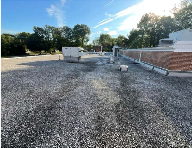
7 - PRIMARY ROOF OVERVIEW
